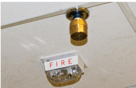
Ceiling-mounted agent discharge nozzle and notification device.
